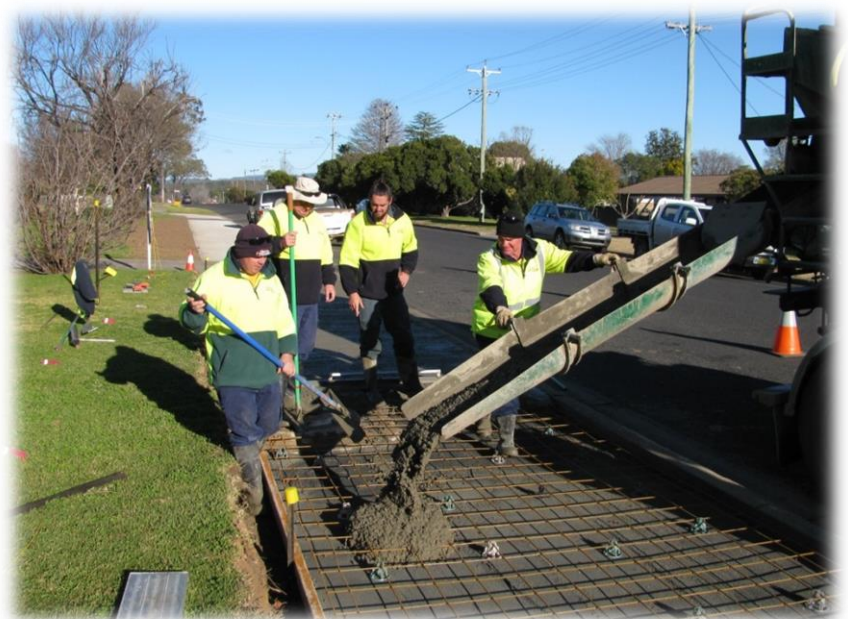
Construction of a new footpath Cassilis Street, Coonabarabran
