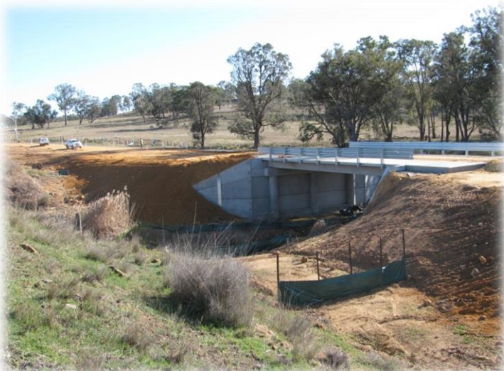
Construction Mow Creek Bridge Binnaway Road
