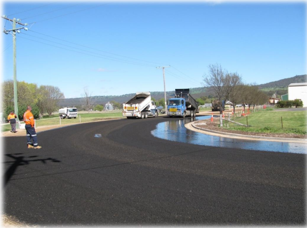
Rehabilitation road pavement Heavy vehicle bypass Coolah
